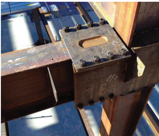
R=3 Completed Connection
