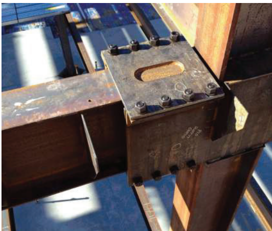
R=3 Completed Connection
